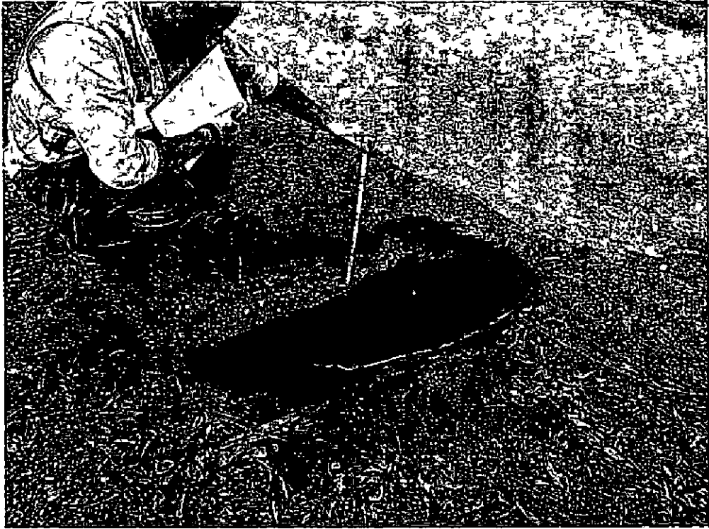
Hole in deck
